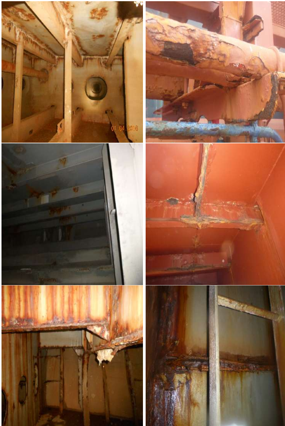
Figure 4.7: Surveys dataset sample of Corrosion class
